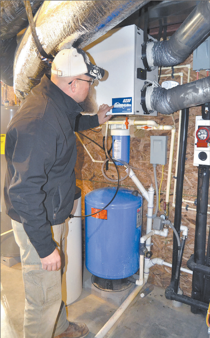
MARY GRZEBIENIAK | Business Chronicle Contractor Pete Mathieu looks over the geothermal heating system. It is only one of several heating options for an Energy Star home, but was a feature that homeowner Jerry Fisher wanted. Geothermal draws heat or coldness from underground using a liquid that is circulated in a closed system of underground pipes.
