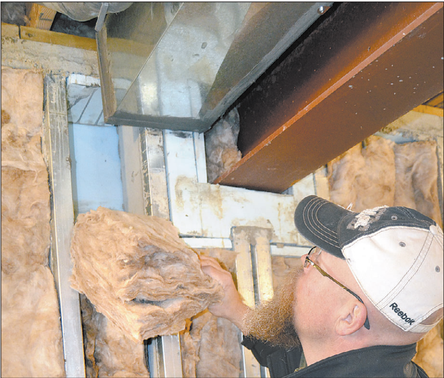
MARY GRZEBIENIAK | Business Chronicle Solid foam behind insulation in the basement helps the house to be 47 percent more energy efficient than the average home.
