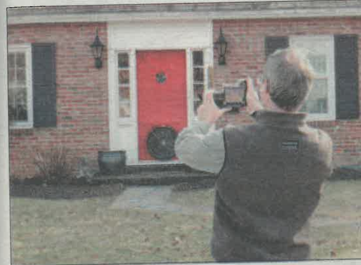
Thermal imaging & a blower door test determine whether a home is built airtight.
